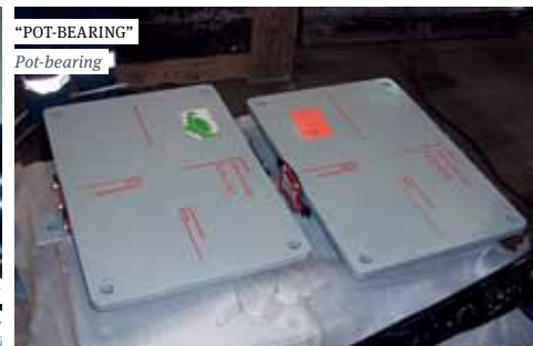
"POT-BEARING" Pot-bearing
