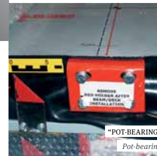
"POT-BEARING" Pot-bearing
